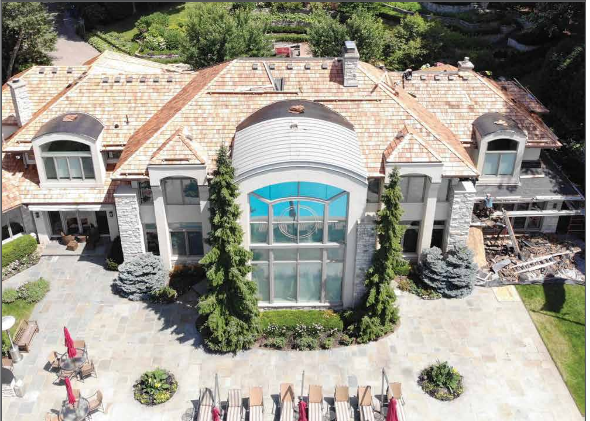
CEDAR SHAKE ROOF REPLACEMENT - ROOF WAS DAMAGED DUE TO HAILSTORM
